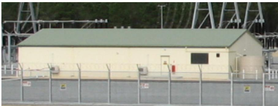
*Standard relay building for 330 kV and 132 kV Terminals*
